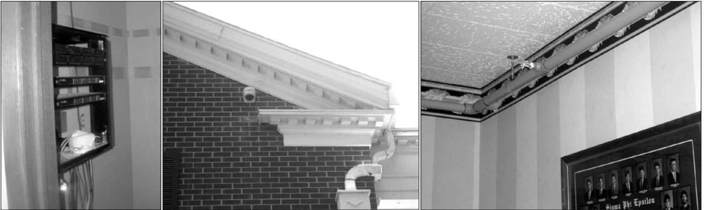
From left: A new mechanical room with a networking service panel for cable, the computer server, and the security camera system; a high-tech security system guards the exterior; and a fire sprinkler system has been installed throughout the house. Below: Work in the boiler room.
