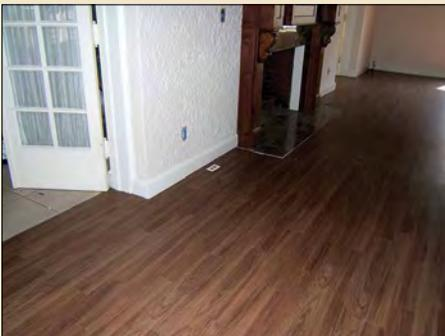
**Left column:** Vinyl plank wood flooring was installed in the east wing corridors and student rooms. The interior was painted and new light fixtures were installed.
